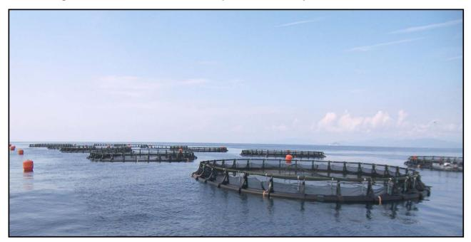
The FUTUR cages are constructed from solid HDPE material throughout. The heavy duty stanchions in 25 mm thick HDPE are stronger than steel counterparts, and provide additional protection against abrasion from boats and heavy farm machinery.
